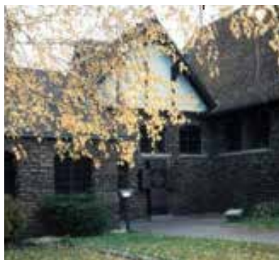
Entrance to the parish hall with the new Columbarium, installed in 1994.
